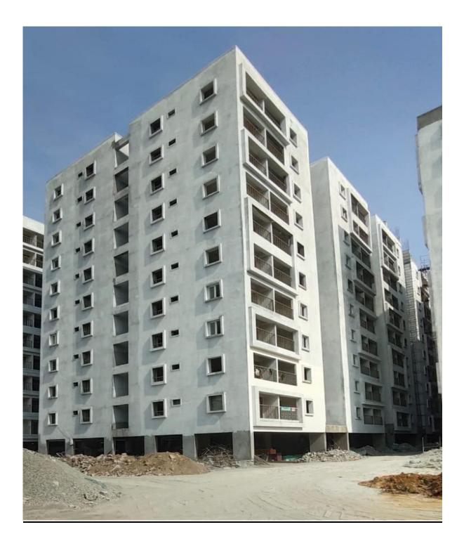
**Block C3:** External Plastering 90% completed. 1st Coat Primer 70% completed.
