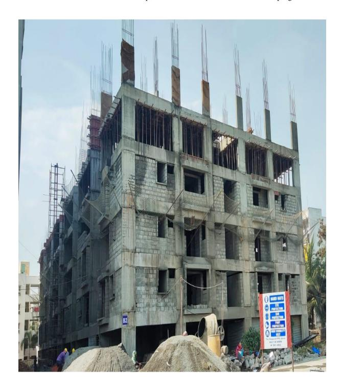
**Block C1:** External Plastering overall 95% completed. 1<sup>st</sup> Coat of Primer 90% completed. Lift Installation works on Progress. Terrace Weathering course work on Progress.
