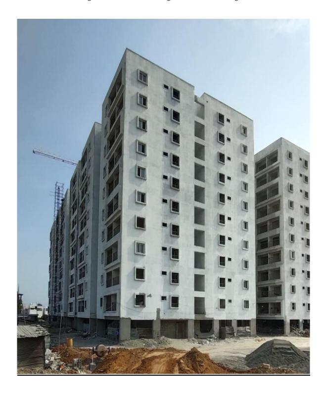
**Block C2:** External plastering overall 95% completed. 1<sup>st</sup> Coat Primer 80% completed. Lift Erection works on Progress.
