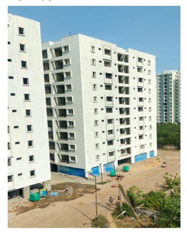
**Block D3:** External Plastering work overall 95% completed. 1<sup>st</sup> Coat of Primer 85% completed. Tiling works on progress.
