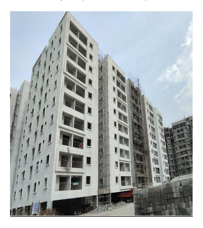
**Block D1:** External plastering overall 85% completed. 1st Coat Primer 70% completed..
